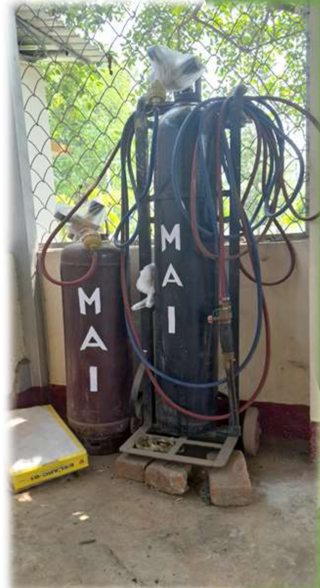
OXYGEN AND ACETYLENE CYLINDERS
